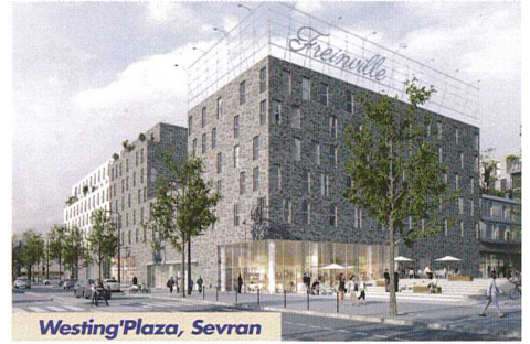
Westing Plaza, Sevran
